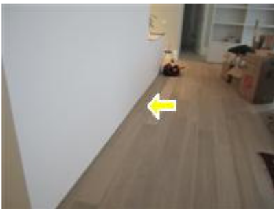
2.6.A Picture 1 living room - no wall receptacles on this wall
