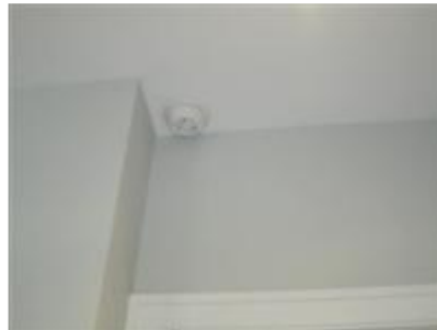
5.7 Picture 1 Heat Alarm - hall area near 2nd bedroom 5.7 Picture 2 dead air space location - not recommended
